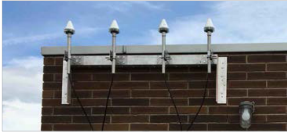
The four antennas mounted on top of the building provide signals from GPS satellites.
